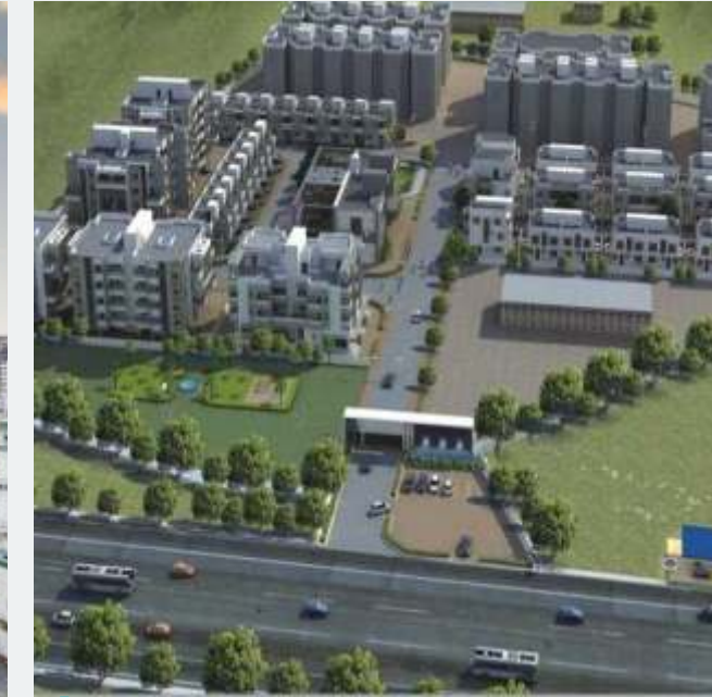
Leverage Greens Constructed around 11 acres
