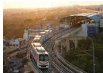
Metro Extension Phase 2*
